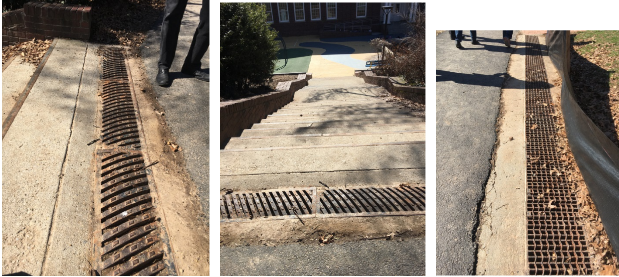
Figure 6. Pictures of sediment and debris deposit at drainage grates
