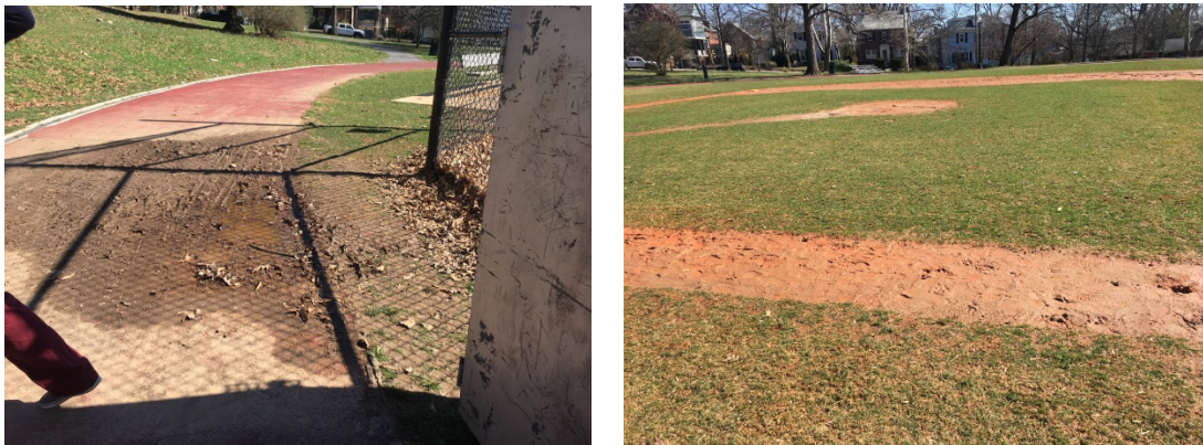
Figure 6. Pictures of sediment and debris deposit at drainage grates
